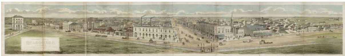
Fig. 3 De Gruchy & Leigh, Panoramic view of Melbourne, Victoria , 1863
