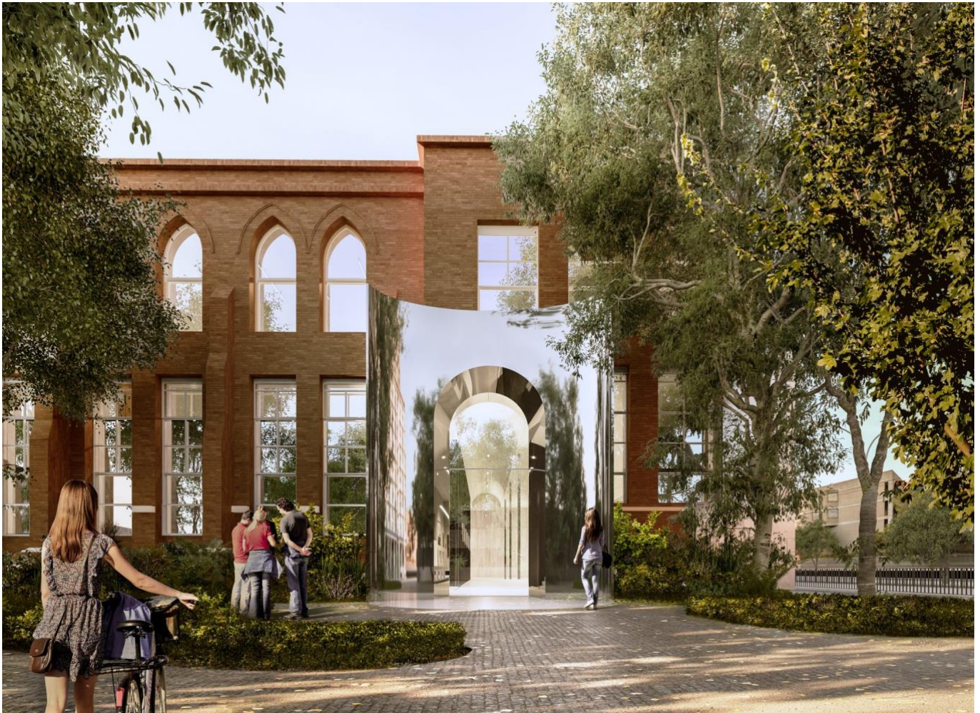
Image: Architectural render of the Potter Museum of Art (The Potter), redeveloped by Wood Marsh Architects.
